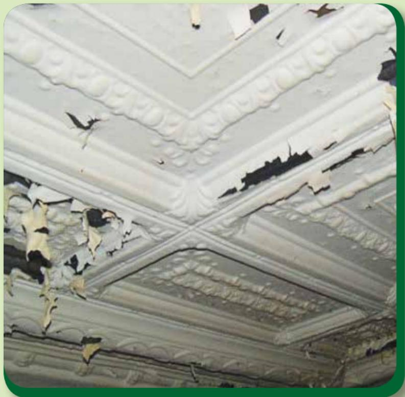
**An image of broken asbestos ceiling tiles**
