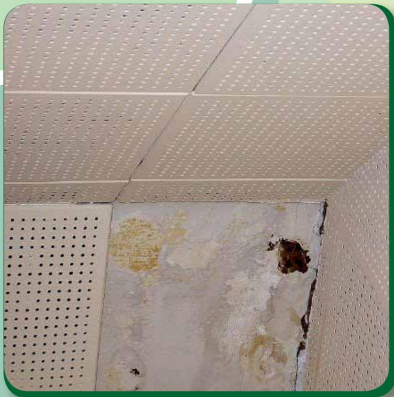
*An image of broken asbestos ceiling tiles*
