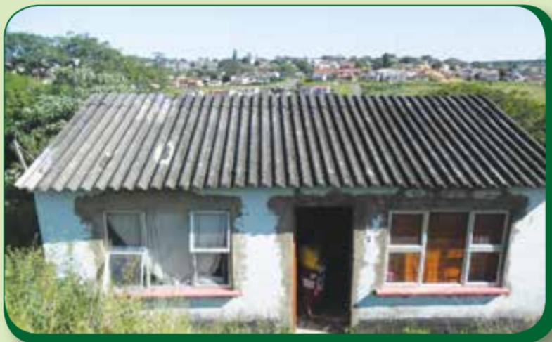
*An image of cement-asbestos corrugated*
