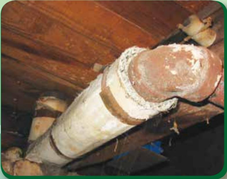
***An image of asbestos used in pipe insulation***
